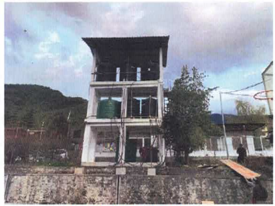
Fig.5: Existing water tanks
