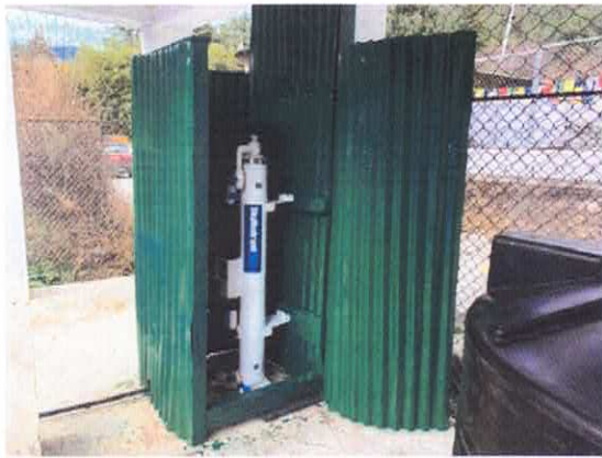
Fig.6: Temporary shed for the filter
